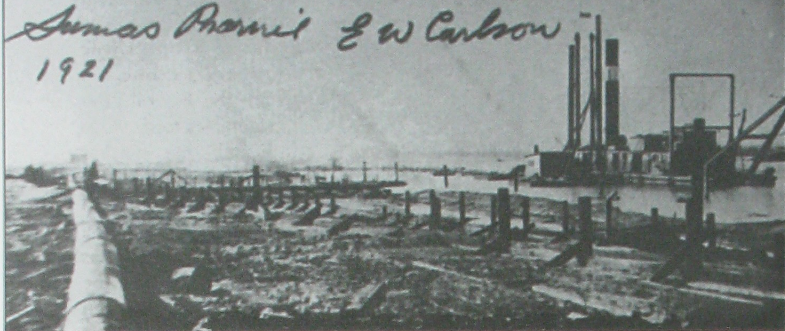
The Sumas Dyking Project of 1878 was merely a prelude for the more extensive activities associated with the Sumas Lake Reclamation Project of 1924. In this photo the dredge "The Col. Tobin" works to dig the Vedder Canal.
